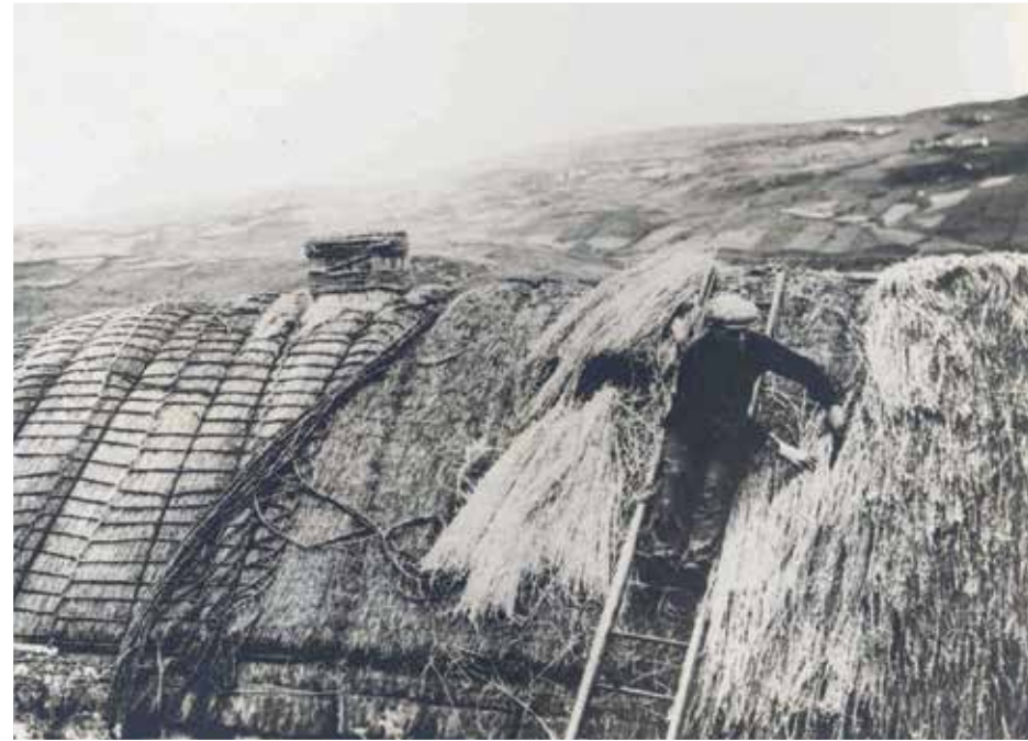
Seamus Ó hEochaidh thatching the roof of a cottage in Rinnakill, Teelin in the late 1930s. The intricate network of ropes [or fishing nets in some coastal locations] that was used to secure the thatch were tied to projecting stones [bacán] at the eaves and on the gables Photograph: Donegal County Archives
